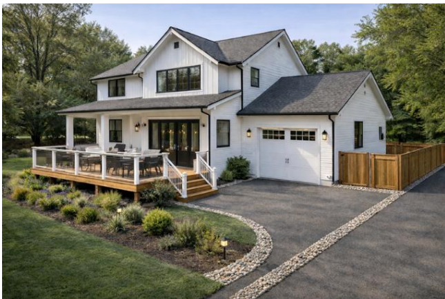
Figure 6. Before-and-after representation of a single-family house that implemented Zone 0. Note the relocation of the plants away from the deck and the installation of a noncombustible gate. While not required, it is best practice to install metal screening around the deck base to keep embers and debris out. Once Zone 0 is finalized, the guidance document will provide tips and tricks for addressing issues like this.
